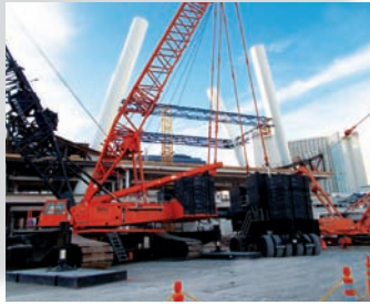
A 2250 Crawler crane (background) is dwarfed by the Liebherr 1750 and its massive counterweight configuration which is required for the critical steel picks
