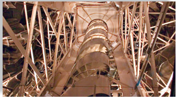
This picture may not be easily recognized as the Statue of Liberty because it is the iconic monument's skeleton!
