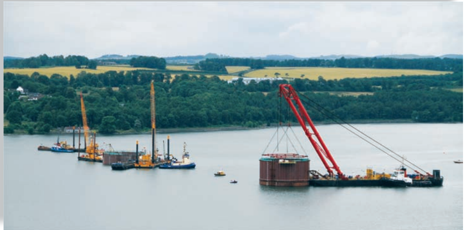
Setting south tower caisson, S1 in back
