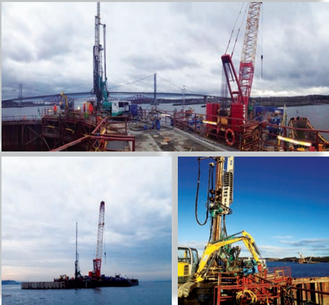
South tower caisson jet grouting and drill rig
