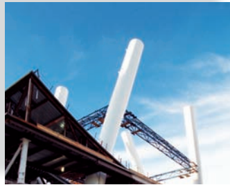
The first of two levels of temporary trusses stabilize the support legs as they grow skyward toward their 282' apex
