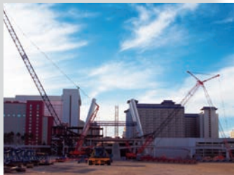
Looking west: the famous Las Vegas strip casinos form the unique backdrop for the structure
