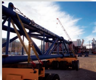
American Bridge dolly system used to transport the temporary stabilization trusses on-site
