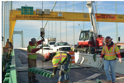
Field Engineer Kara Mullin watches as AB Ironworkers set new finger joint section at the NJ tower, using a 15 ton Tadano crane
