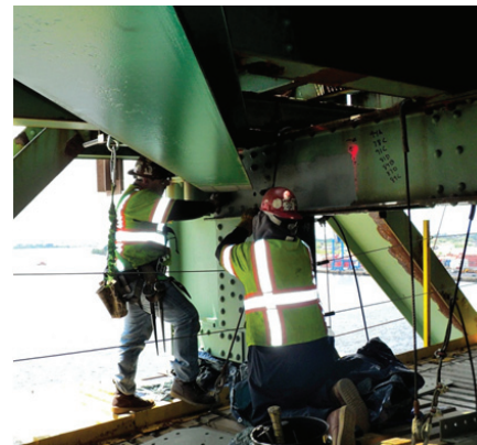
Ironworkers installing new top lateral bracing members during the advanced work stage from the temporary work platform
