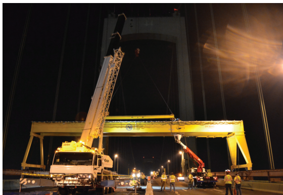
Superintendent George Terrance and General Foreman Mike Rambus oversee erection of the 86'-8" gantry crane box girders; AB set the six girders during one, four-hour, full-bridge shutdown
