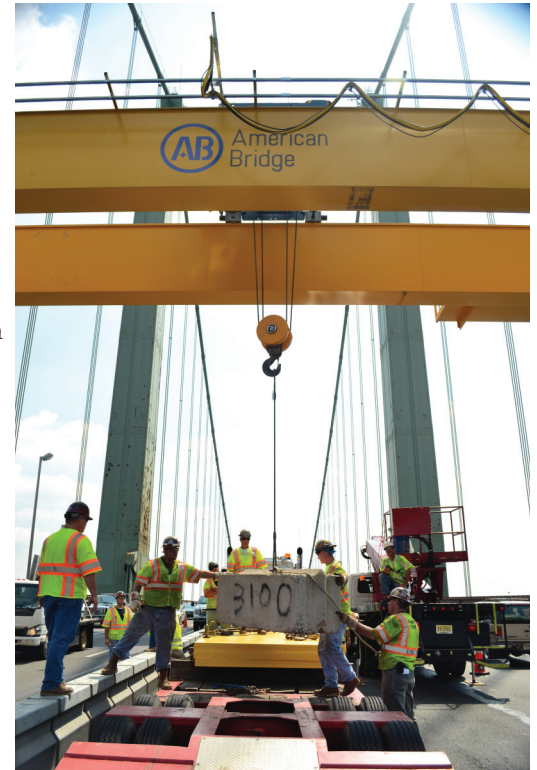
George Terrance and Mike Rambus oversee gantry load test
