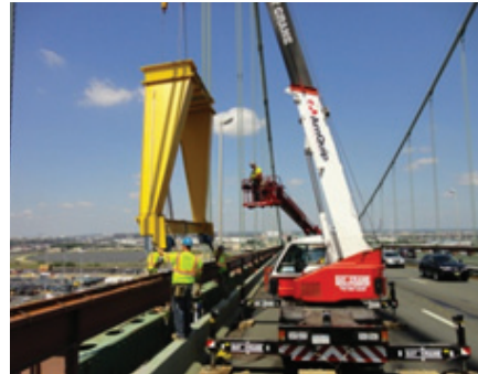
Erection of the gantry crane legs with the 15-ton Tadano crane
