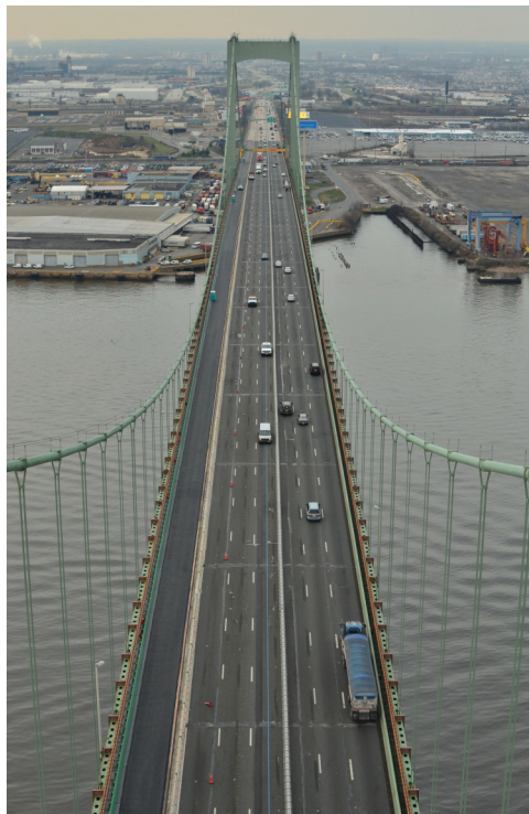
View of the new deck (Stage 1), as seen from the top of the NJ tower
