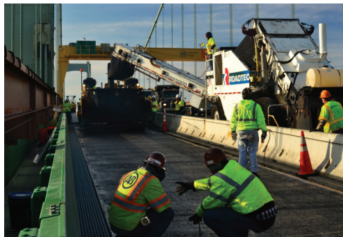
Field Engineers Michael Hartranft and Drew Merritts examine the new deck as workers pave Rosphalt overlay
