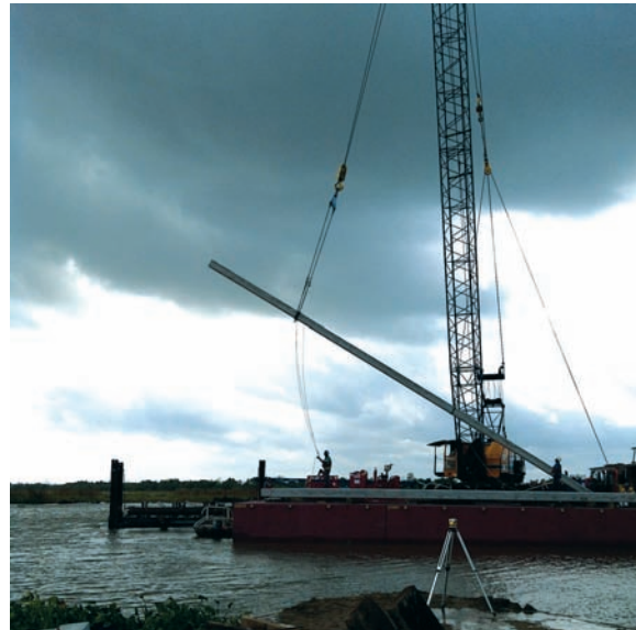
Handling and driving of such slender and long piling with limited access off a major highway
