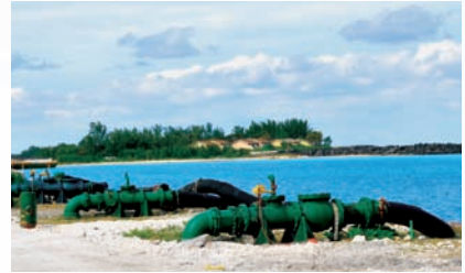
Permanent water system to be relocated
