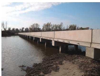
West Bridge, currently 95 percent complete
