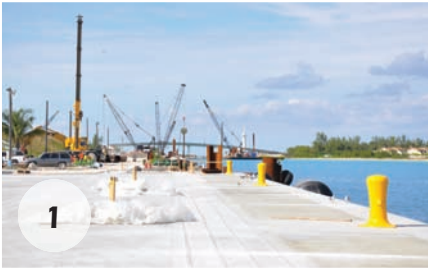
1 The contract required the first section of the port to be complete by November 30th, 2010 to allow container terminal operations to relocate from its western-most location at the port, enabling AB to start work in that area keeping ahead of schedule
