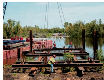
Crew setting template through which prestressed concrete piling are driven
