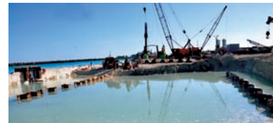
Sheetpile, high tide
