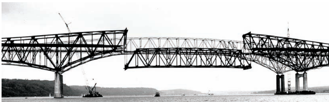
AB erecting the 500' long, 1,800 ton truss assembly to complete the superstructure framing for the second Newburgh Beacon Bridge in 1980 (This is Crossing the Hudson's cover image provided by American Bridge archives)
