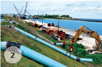
2 Temporary water system
