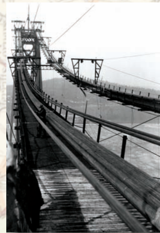
AB's cable spinning made from airspun parallel wires for the Mid-Hudson Bridge in 1928
