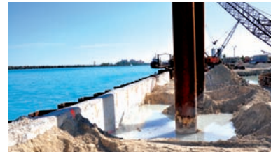
Some of the piles could not permeate the ground's hardness so the design was changed, set of piles every 10'
