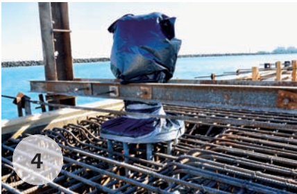
4 There will be twenty-nine 100 ton bollards along the replacement wall
