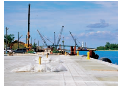
Completion of the first pier section was required by November 30th, 2010 in order for one of the tenants to relocate all of its equipment
