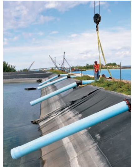
Temporary water system pouring into reservoir
