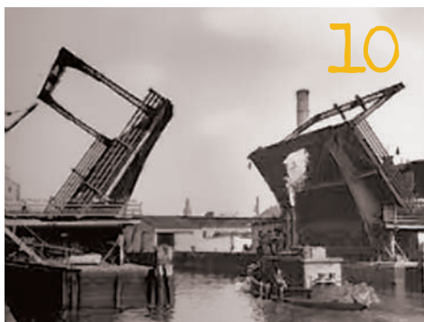
9th Street Bridge Location: Brooklyn, NY AB employees:
