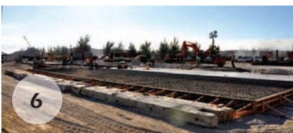
6 Frame with rebar for concrete deck
