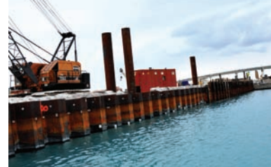
American Bridge is constructing 2,500LF of new sheetpile bulkhead with concrete encapsulation
