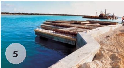
5 Construction of two concrete encapsulated, pipe pile supported RORO docks
