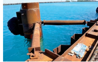
AB created temporary fendering system allows the crew to continue construction while ships unload
