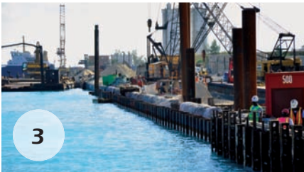
3 Existing wall and piles with rising tide
