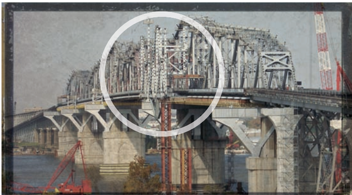
The Huey P. Long Bridge is being widened to increase the number of North and South bound traffic lanes by the addition of new outside trusses connected to the existing structure by new floorbeams, struts, portals, sways and laterals. This widening will occur on both sides of the existing bridge
