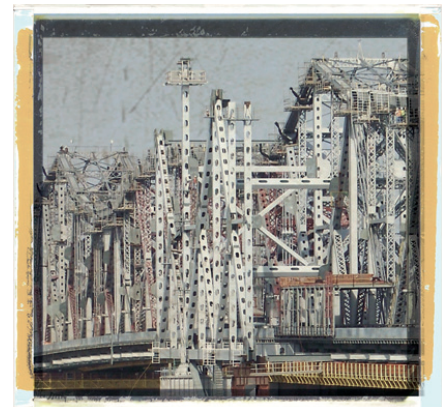
The start of erection on one of the two new trusses along with the widening members. Erection will continue along each side of the truss bridge throughout 2010 and into early 2011
