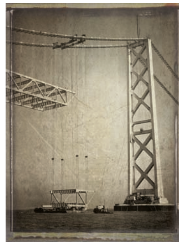
Truss lifted from barge
