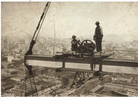
Men working with Derrick Swing Winch 1935
