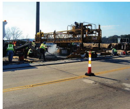
LMC placement on the eastbound traffic lanes
