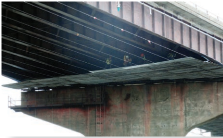
Painters installing under the structure platform
