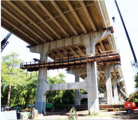
Raising jacking platform for sole plate and bearing replacement
