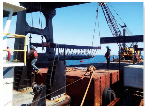
Setting gabion baskets tandem pick American 5299 and Manitowoc 4100
