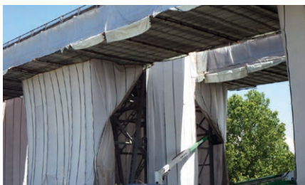
Overall view of truss span
