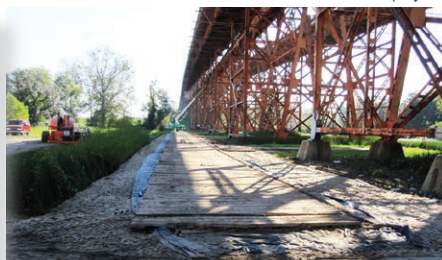
Crane mat access road
