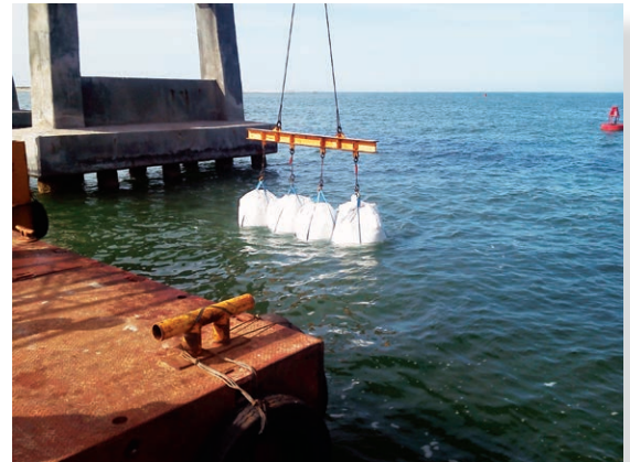
Installing the last sand bags
