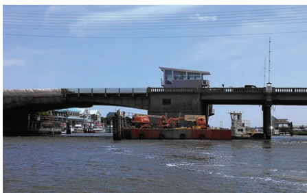
Containment platform installed on the far leaf to support cleaning and painting operations
