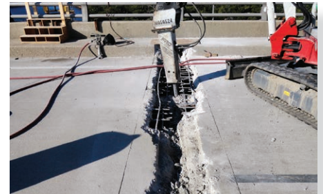
Deck joint removal and replacement
