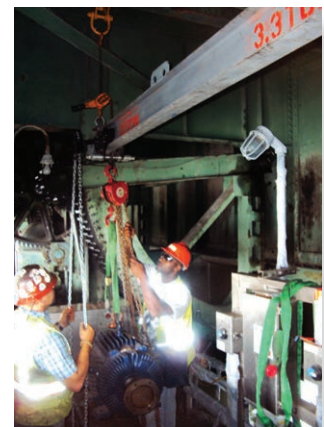
Staging machinery components on the machinery platform for replacement
