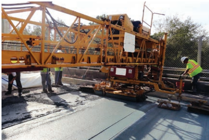
Placing latex overlay
