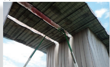
Bent containment with lifts to railroad girders
