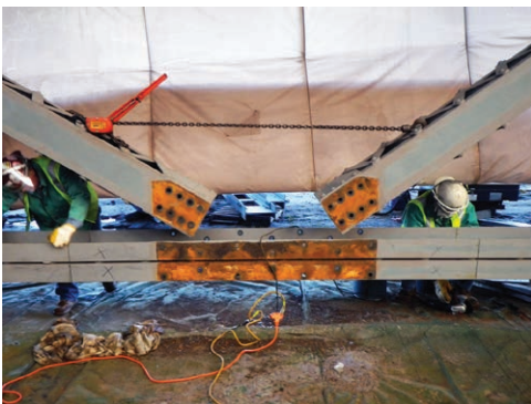
Bottom highway horizontal member replacement
