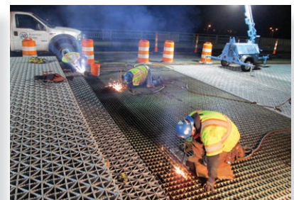
Crew removes existing grid deck welds by air arc gouging
