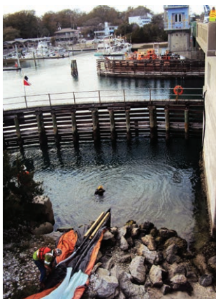
Crew pulling three new submarine cables across the intracoastal waterway
