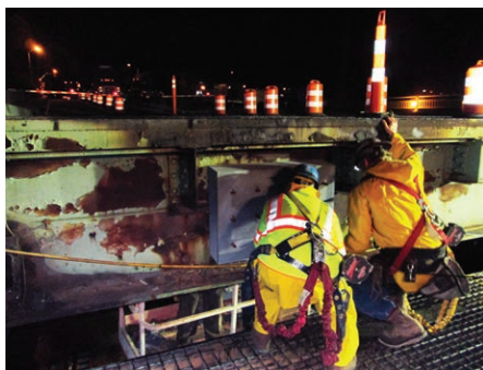
Span balance adjustment utilizing steel balance plates installed at the span's toe
