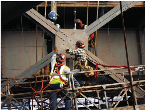
Railroad tower diagonal bracing replacement
