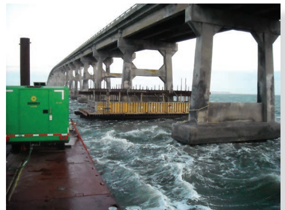
Strong currents preventing access to bent 159 cap and dive work
