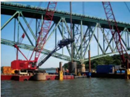
Drilled shaft installation
