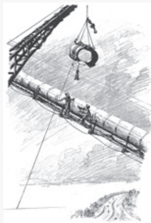
Cable band being lowered into position, Brooklyn Belt Parkway below, 1963
