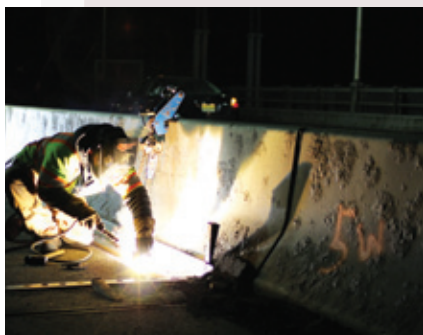
Welding the newly installed curb angles on the existing deck using beam clamps (shown in the median) to change the elevation of the angle, as the back side of the angle is floating on air until it is welded
