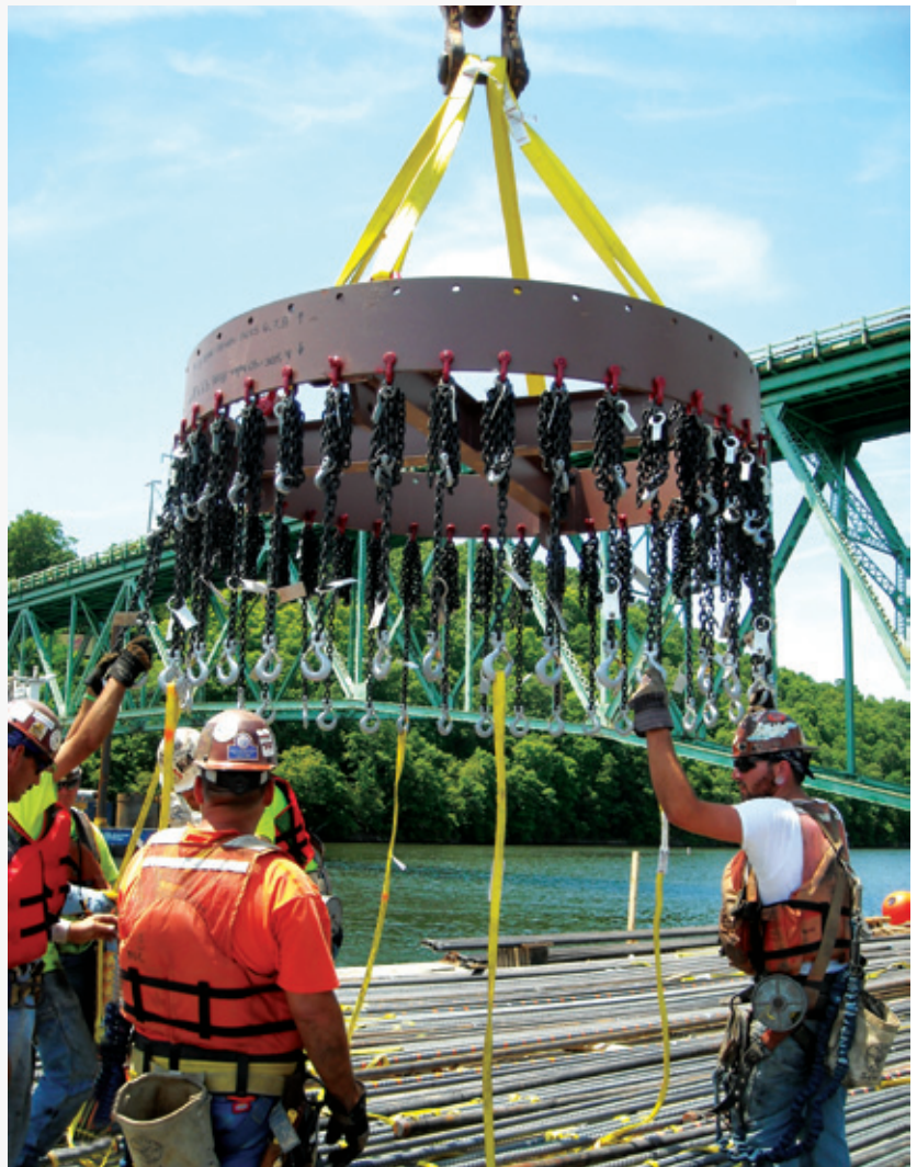
Wind chime reinforcing cage rigging
