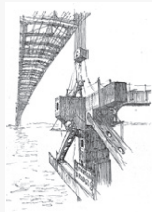
Four-hundred-ton center span roadway unit near Brooklyn tower, 1964
