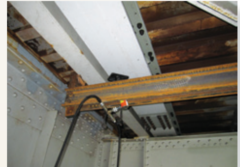
Secondary floorbeam jacking system to raise the beam to make the connection to the existing deck
