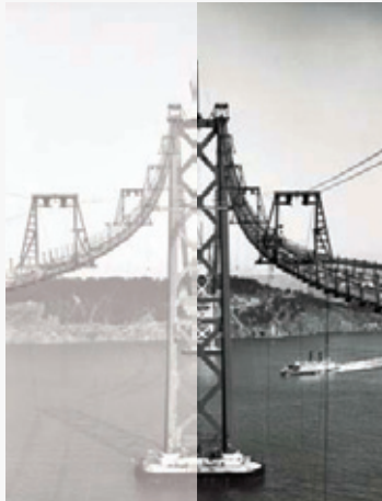
Built original east and west span 1935
