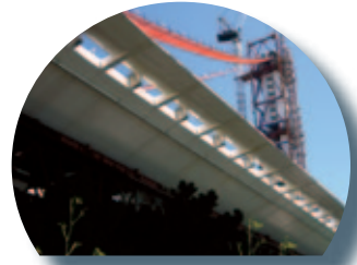
Each of the two 182.9m (600') long side span catwalks weigh 23.6 mt (26 tons)
