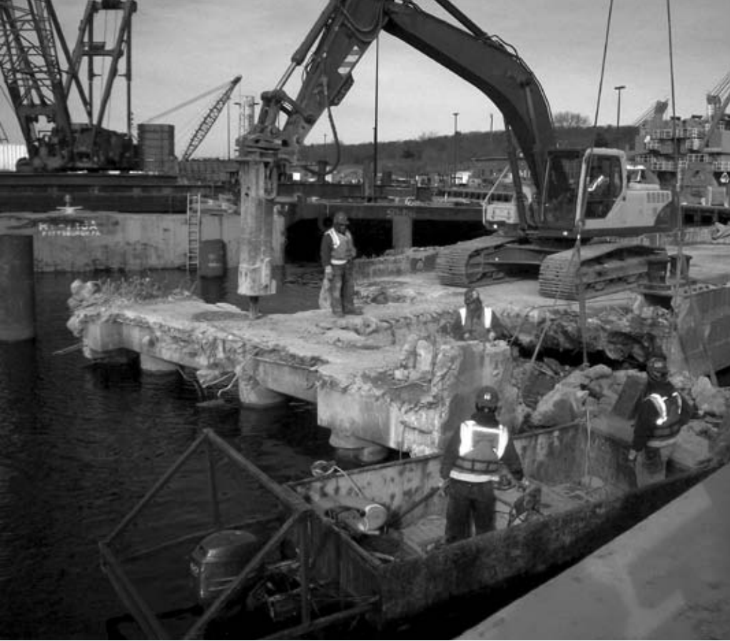
Work began with the demolition of the old Pier 31
