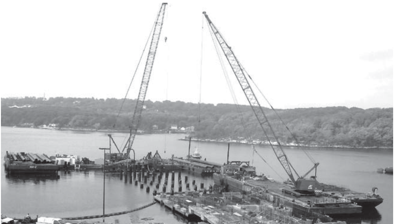
Pier 6 Replacement was one of dozens of projects from which AB drew to meet the challenges of Pier 31
