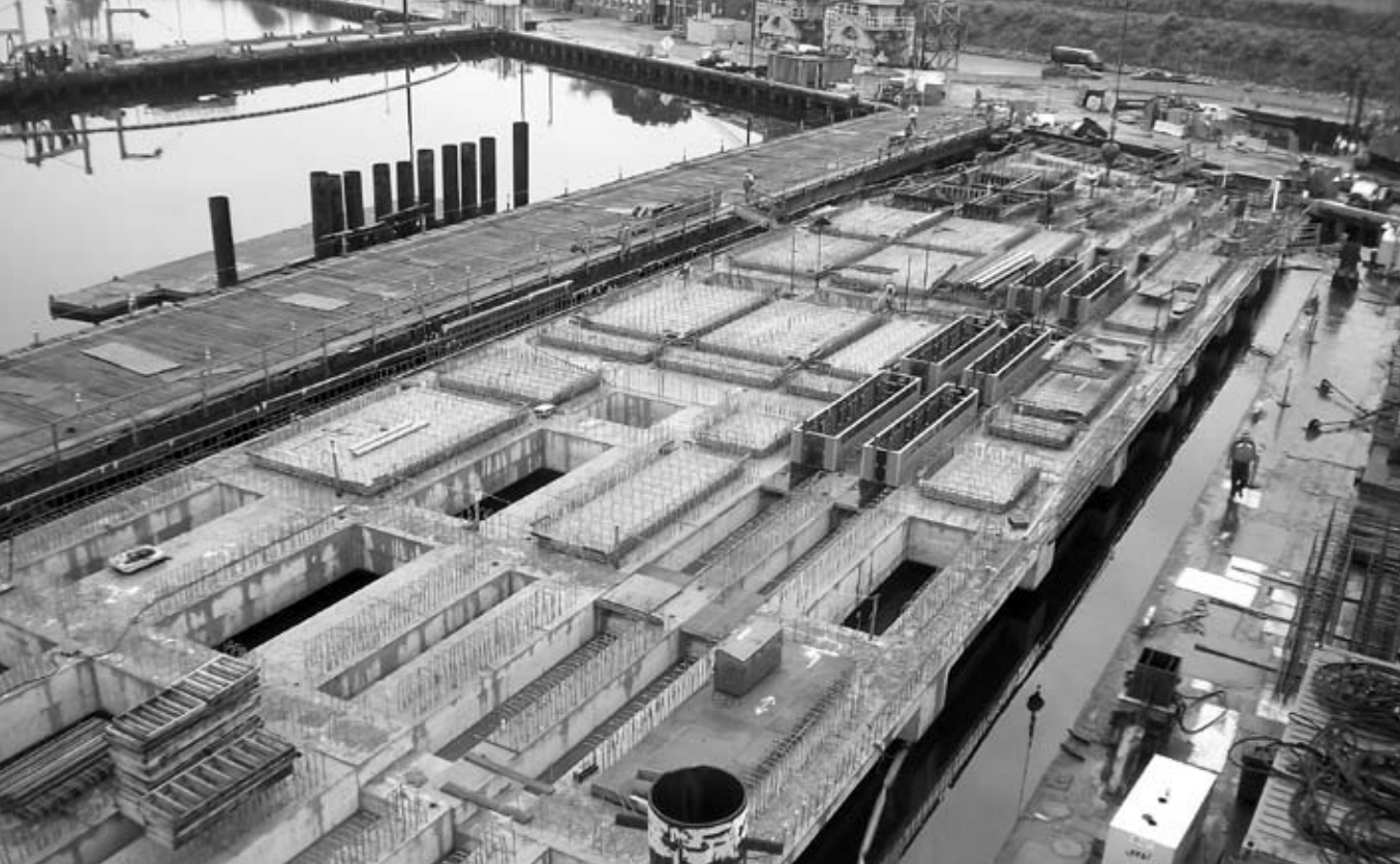
Pier substructure concrete completed from bents 1 to 21
