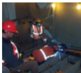
FCAW-G weld made from the inside
