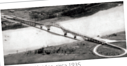
Southbound bridge, circa 1935
