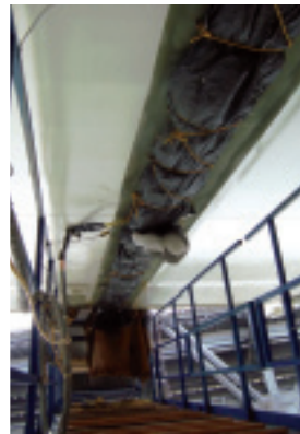
HEAT BLANKETS insulation installed on the outside face covering the joint and fit-up-gear
