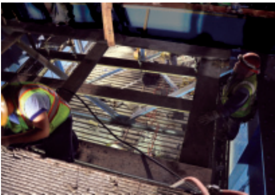
Wood planking for temporary access in order to clean & prepare the existing steel floor beams
