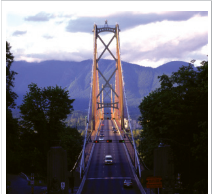
Lions Gate Bridge, Vancouver, British Columbia, Canada American Bridge design-build contract
