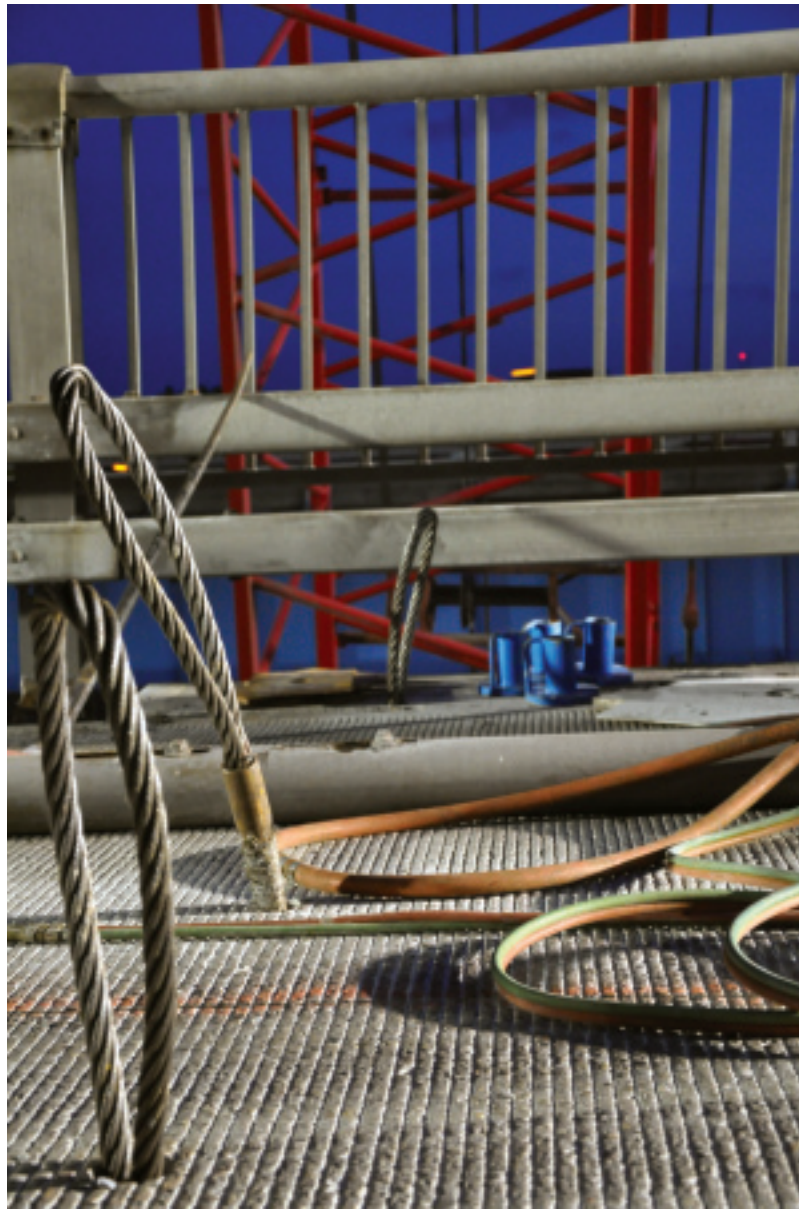
Existing deck of the northbound South Grand Island Bridge waiting to be lifted by the red crawler crane using the gray-metal rigging and blue teacups
