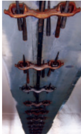
ANCHOR the backing bar with fit up gear
