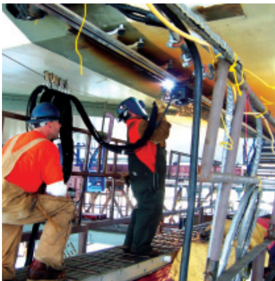
BOTTOM PLATE is accessed from the typical truss crosswalk
