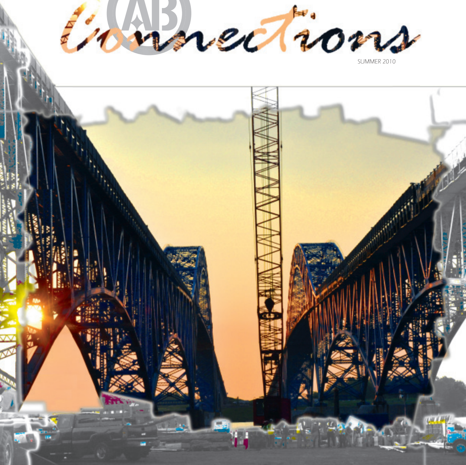
SOUTH GRAND ISLAND BRIDGES New York Historic Landmarks
