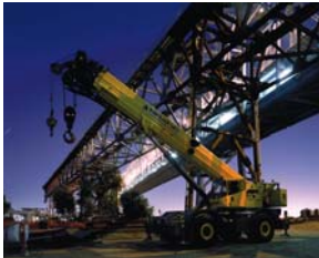
Mating of the OBG in fabricators yard
