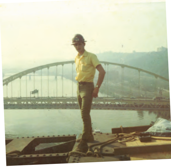
Dan standing atop the Manchester Bridge during demolition in 1970
