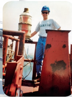
Murphey atop the Tagus Bridge Tower before AB work commenced
