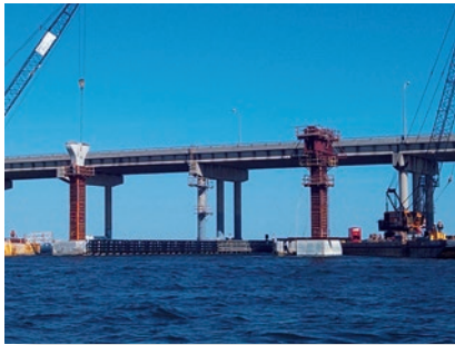
Column and pier cap construction at mid-span
