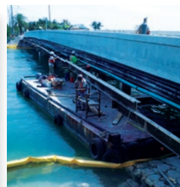
Crew installing 4" force main after completion of east bridge deck
