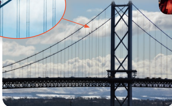
Birds-eye-view and close-up of the main cable walk
