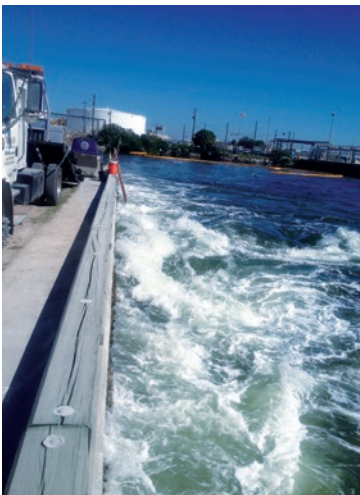
Typical assist-tug prop wash influence on bulkhead
