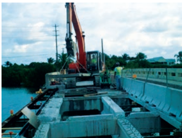
Demolition crew removing deck slab on east half of bridge
