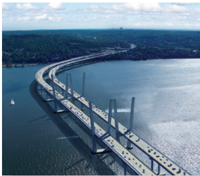
Renderings of the new Tappan Zee Bridge
