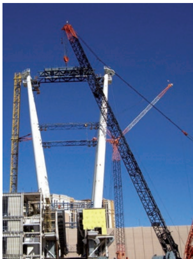
Hub and spindle truss
