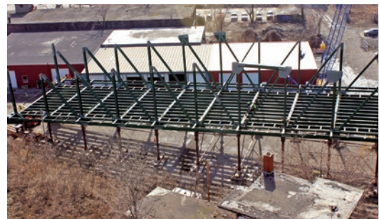
Top of Carter Road Lift Bridge during top chord installation (photo: Wes Weir Transystems, 2013)
