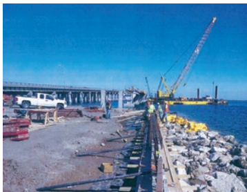
Sheet pile cap formwork; MSE wall construction; rip-rap placement in coffer cell
