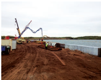
Placement of upper portion of the concrete cap in the foreground; completion of clamshell dredging in background
