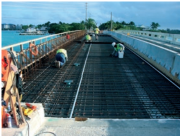
Crew preparing for first deck concrete pour after formwork and rebar has been installed
