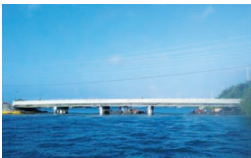
East half of the bridge completed with sidewalks and traffic railing; crews removing formwork and installing handrails
