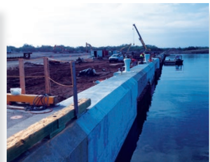
Progress on the concrete encapsulation to date including the bollard installation
