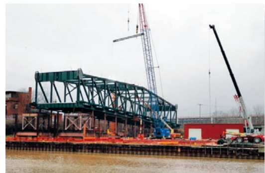
Truss during sway bracing erection; Puerto Rico falsework and pile can be seen at the end of the bridge closest to the river
