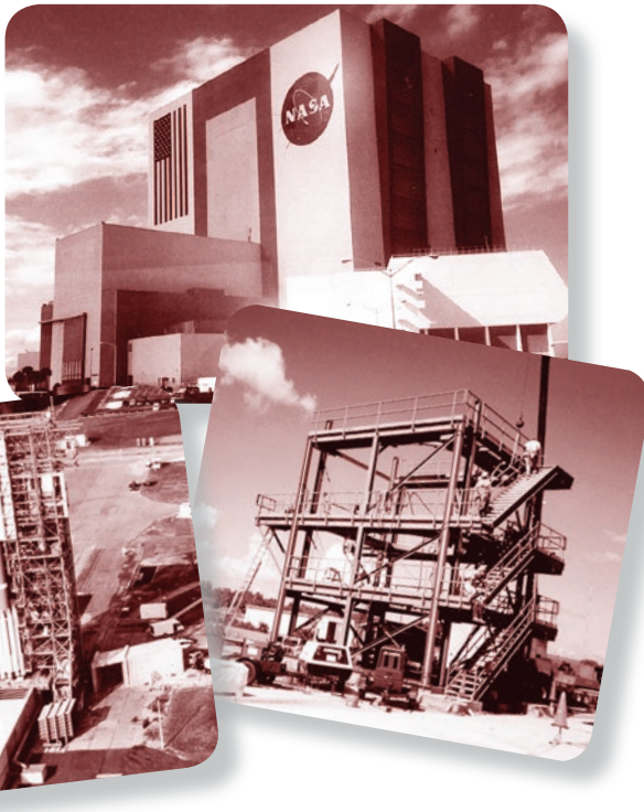
Clockwise from top: Vehicle Assembly Building, Kennedy Space Center, FL; Boeing Delta III 2 nd Stage Test Stand, Cape Canaveral Air Station, FL; Boeing LC 17B Modifications, Cape Canaveral Air Station, FL
