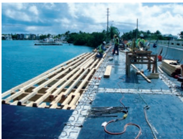
Crew installing formwork in spans one and two
