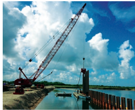
Crane installing sheet piles on a pipe-z combination wall after the pipe piles have been installed
