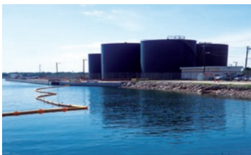
Turbidity curtains deployed ahead of soil excavation; looking back at existing wall; tie in demolition can be seen in the distance
