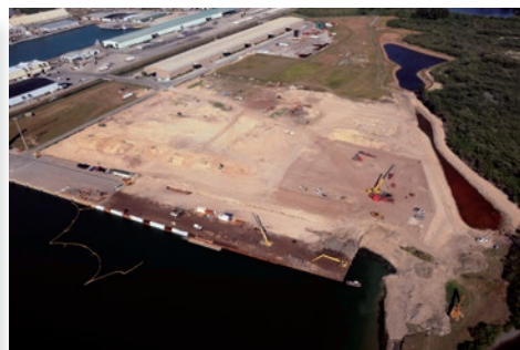
Concrete encapsulation underway on the bulkhead, the newly expanded drainage pond, subgrade work on the container yard and preparation for the installation of a shoreline protection system in the lower right hand portion of the photo
