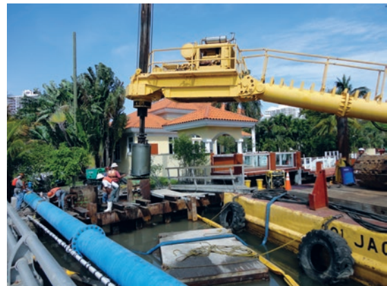
Drilled shaft
