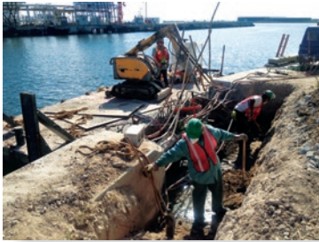
Demolition of the existing concrete cap where the new bulkhead ties into the existing bulkhead
