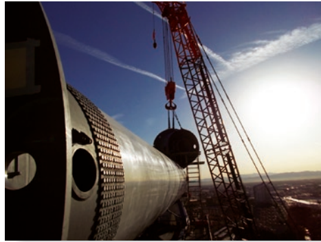
Hub and spindle erection
