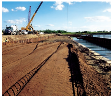
Installation of the tieback system comprised of tierods anchored in concrete inside of the bulkhead pipe piles and connected to a sheet pile deadman wall
