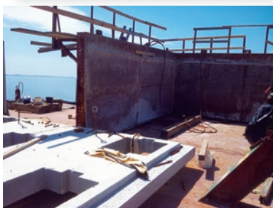
Preparing forms; form and seal grouted in place; completed pile caps
