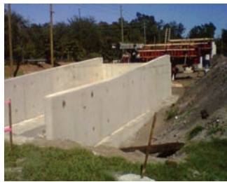
South cantilever wall complete
