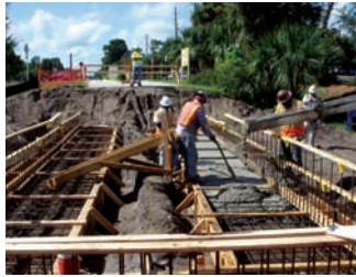
South cantilever wall footer being placed
