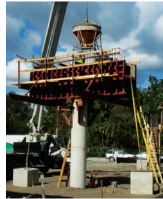
Concrete placement at pier cap six
