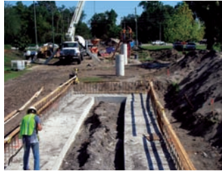
South cantilever wall footer complete
