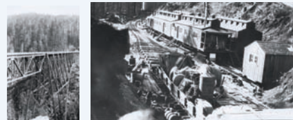
Vance Creek Bridge
