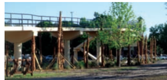
South side with handrails and landscaping in place
