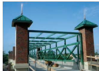
Pier eight entry to the mainspan nearing completion
