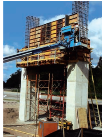
Installing pier seven beam form work
