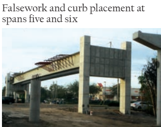
Mainspan precast beams in place
