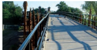
South approach awaiting fence fabric installation
