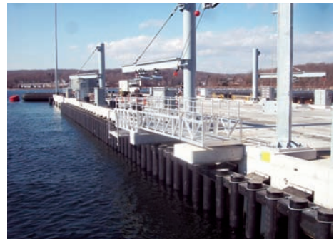
South side of pier
