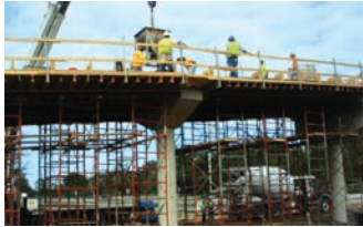
Falsework and curb placement at spans five and six
