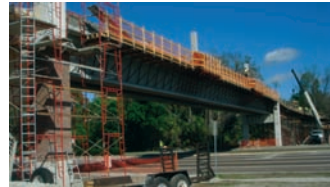
Temporary mainspan work platform and decorative brick installation at pier seven
