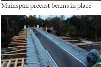
Installing stay-in-place forms on mainspan precast beams
