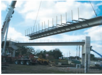
Setting precast beams at span seven
