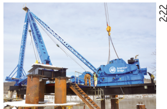
Install 35 kip hoisting engine
