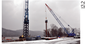
Upper pile driving
