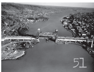
Project name: Portage Lake Lift Bridge Location: Houghton/Hancock, MI AB order no.: V-1662
