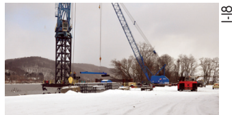
First derrick sill erection
