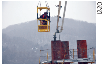
Filling piles with concrete
