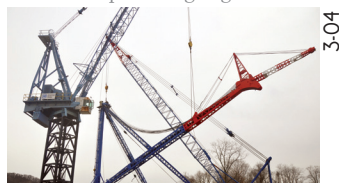
Installing boom and reeving the mast
