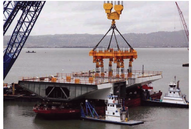
LCL beings to lift 1W
