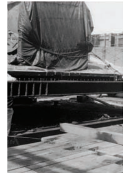
Grillage and base before jacking operation
