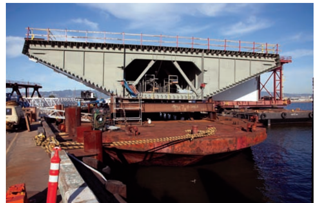
OBG's were unloaded and placed onto 72' x 250' x 15' barges
