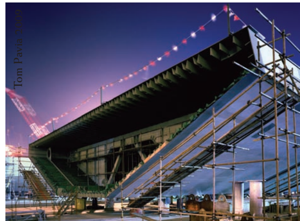
An OBG manufactured and pre-assembled in Shanghai, China
