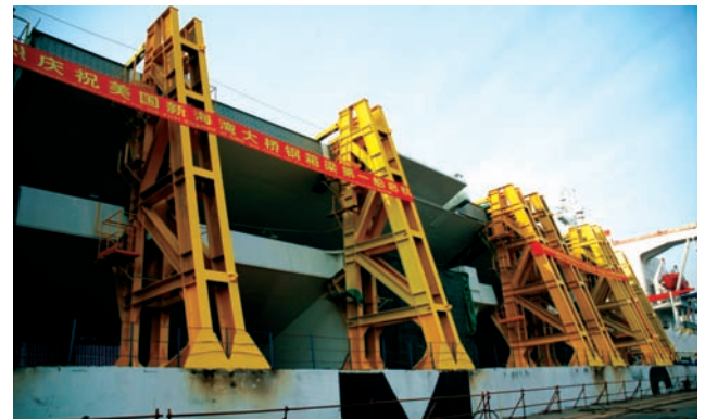
Shipment arrives at ABFJV dock held in place by 30mt sea fastenings
