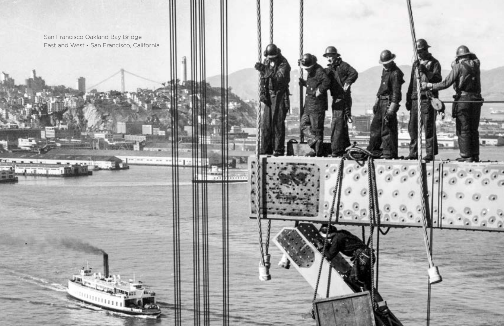
San Francisco Oakland Bay Bridge East and West - San Francisco, California
