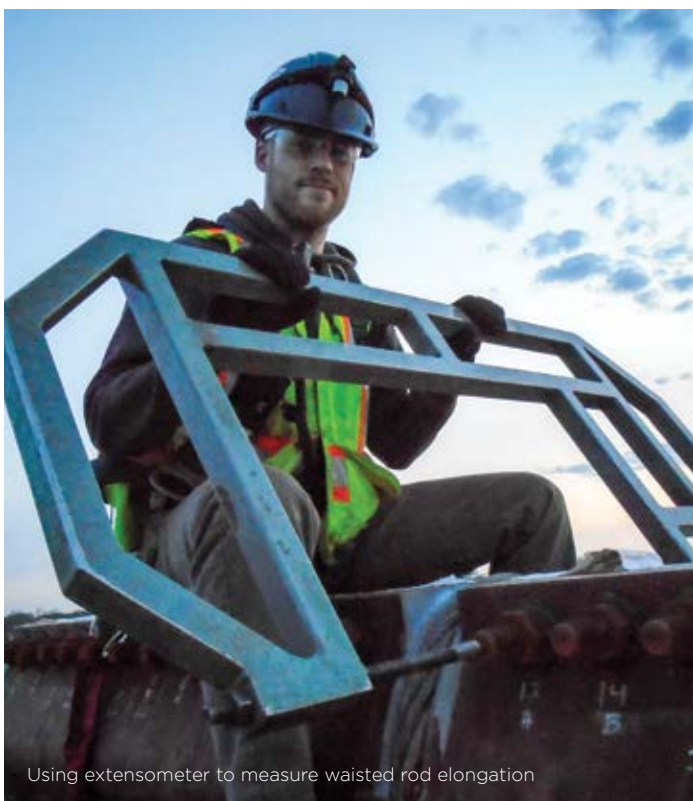
Hanger jacking assembly marked for span raising
