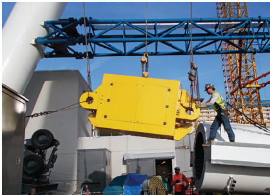
One of eight temporary hydraulic gripper-boxes is mounted onto first rim segment
