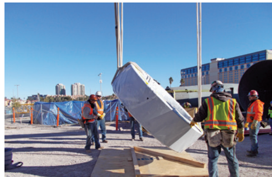
One of 12-ton main bearings, some of the biggest in the world, are unpackaged and 'tripped' upright ahead of installation onto spindle
