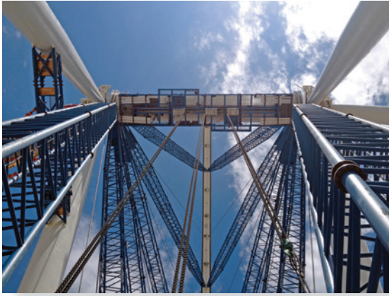
Looking upward at array of temporary radial struts that hold rim in position as it is pushed up and over the hub
