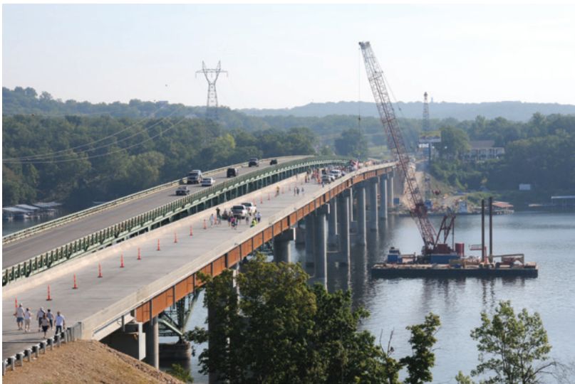
Overview of bridge
