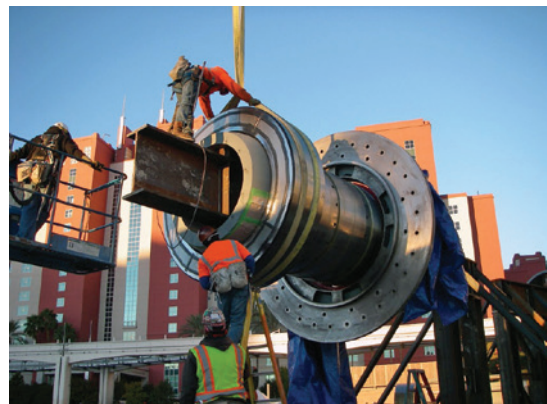
Installing first bearing onto spindle
