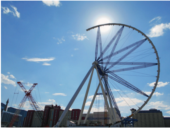
Partially completed rim with Las Vegas Strip in backdrop
