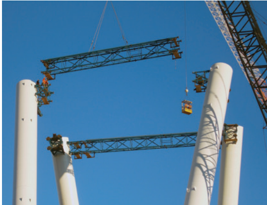
One of eight temporary stabilization trusses is installed between legs
