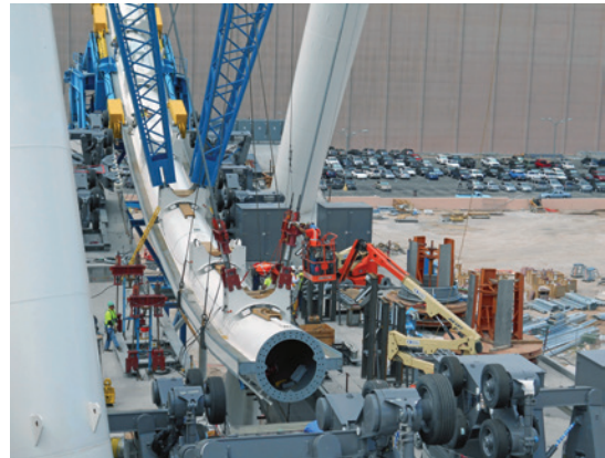
Ironworkers use 100-ton jacking frames to attach 3" diameter locked coil cable spokes to partially completed rim
