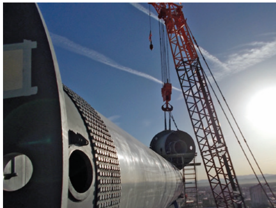
Liebherr 1750 hoists east hub and spindle assembly to elevation 280' above ground
