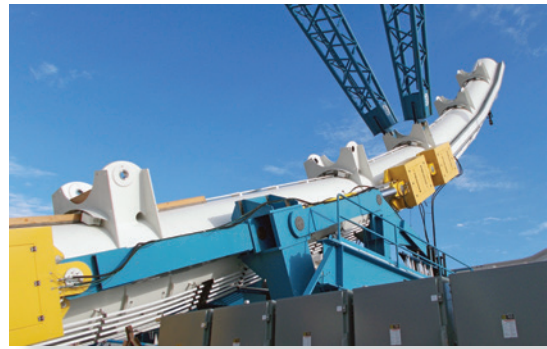
First three rim segments protrude from 750-ton capacity temporary hydraulic rotating mechanism
