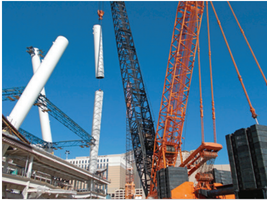
Liebherr 1750 lifts 60-ton leg section into position
