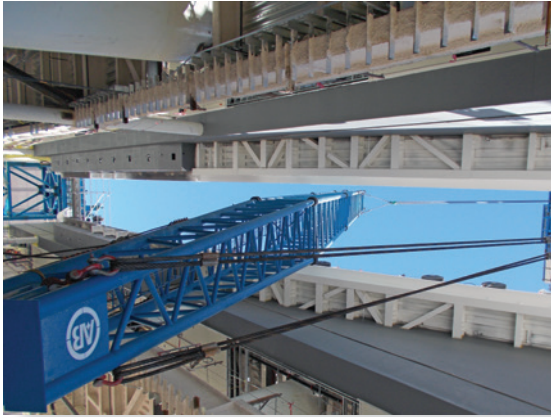
First 40-ton temporary radial strut is hoisted to the hub
