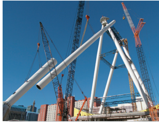
Liebherr 1750 hoists 172-ton upper section of brace leg into position while a lattice boom truck crane suspends the 52-ton lower section
