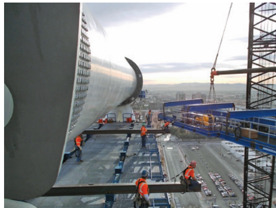
Local 433 ironworkers await perched 265' above Las Vegas on temporary dunnage beams ready to guide chain fall platform into position
