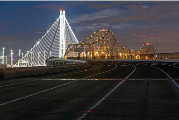
View of the new east span and the west span (completed by AB in 1936)
