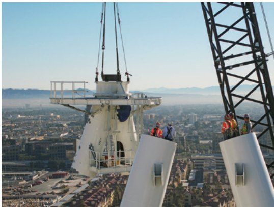
Local 433 ironworkers wait in position in upper legs as east 'pant' section is raised to elevation
