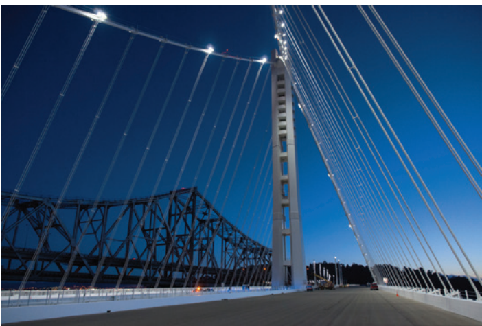
New east span SAS
