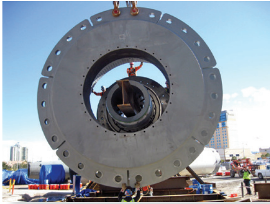
The 134-ton hub is installed over outer collar of bearing
