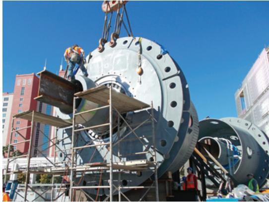
East and west hub and spindle assemblies await installation
