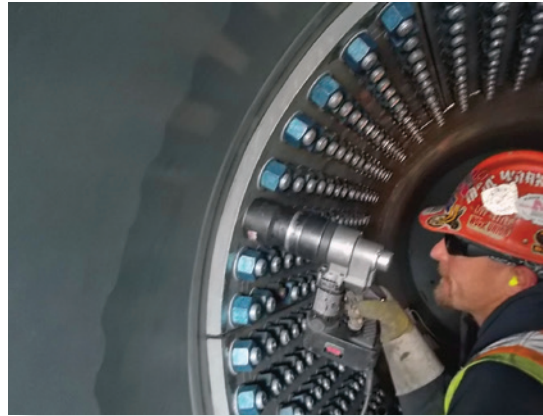
Ironworker shows the ease of using TN33 electric torque wrenches which enable increased production and reduce noise inside spindle
