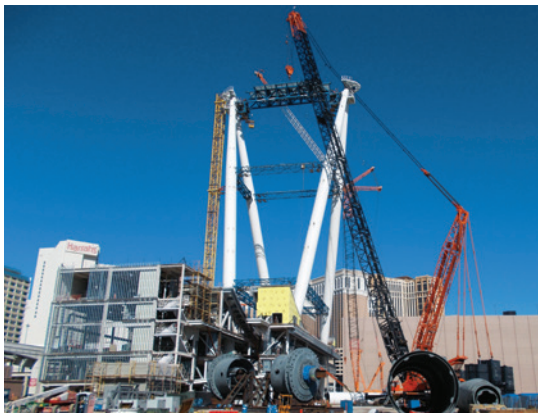
Temporary hub and spindle transfer truss is installed at the top of the support legs 180' above ground
