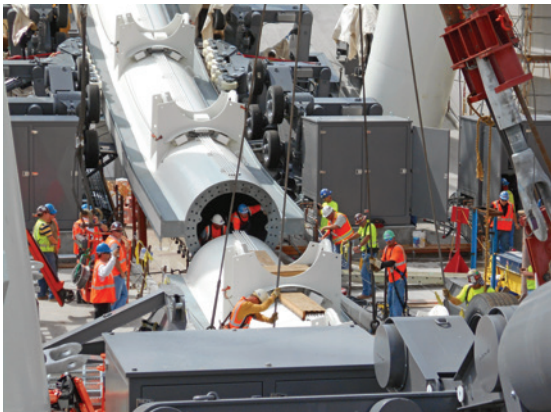
Final rim segment installed and wheel rim is officially closed
