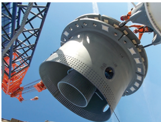
The 177-ton assembly is carefully lowered onto end casting before making inner splice
