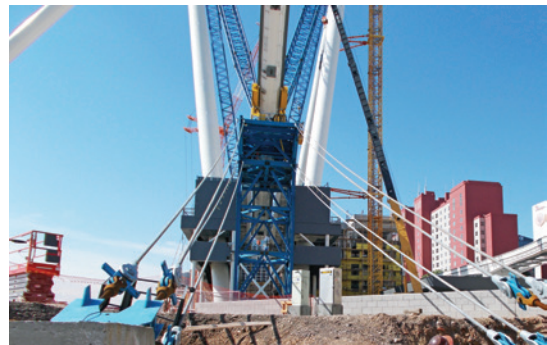
An 80' tall temporary holdback tower with 2.5" stay cables is used to resist eccentric load of partially erected wheel rim
