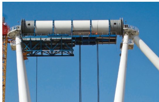
Two of the 55-ton capacity air hoist chain falls lower 40-ton east section of transfer truss out of structure
