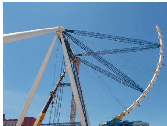
Hydraulic rotating mechanism pushes leading edge of rim upwards as new segments are added at the bottom
