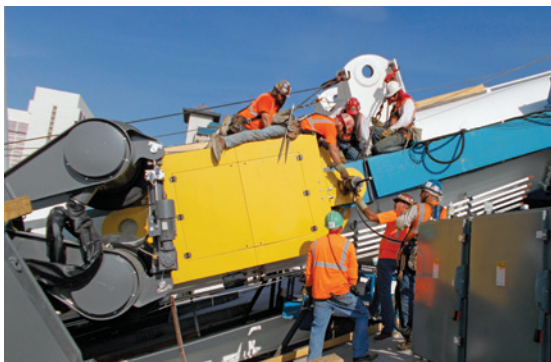
Ironworkers connect lower gripper-box to link arm as the temporary hydraulic rotating mechanism comes together
