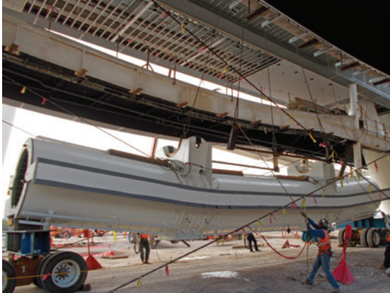
First of 45-ton rim segment is rolled into position directly under legs as hub mounted chain fall is rigged for lifting
