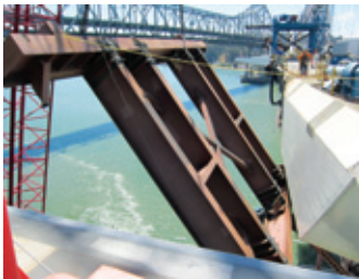
Cradle 14E being tripped up using a barge mounted Series-3 Ringer, as seen from above
