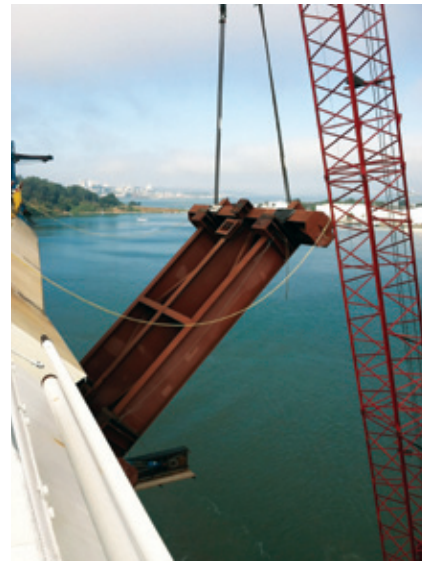
Cradle 13W being pulled out from underneath the bridge; San Francisco in the background
