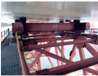
Cradle 13E loaded, prior to removal
