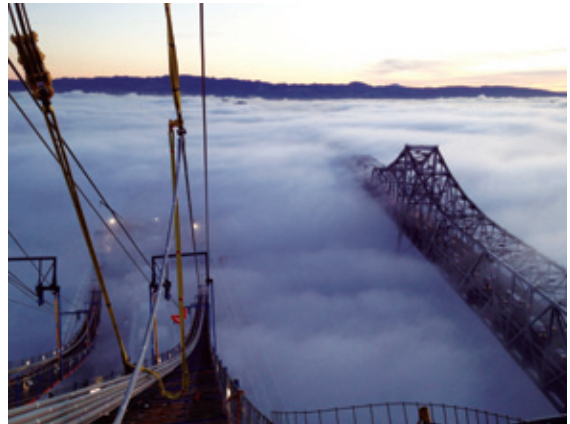
San Francisco/Oakland Bay Bridge Self-Anchored-Suspension Span by Zach Lauria
