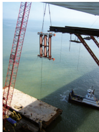
Cradle 13W being lowered to the scrap barge
