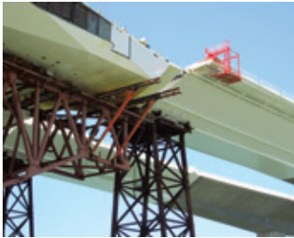
Removal Beam setup under eastbound OBG
