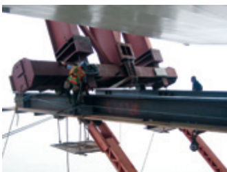
Cradle 13W being tripped up with barge mounted ringer
