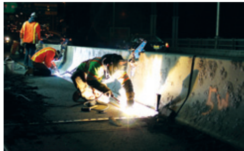
Walt Whitman Bridge - Suspension Spans and Anchorage Spans Deck Replacement by Bruce Phillips
