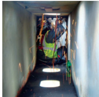
Sherman Minton Bridge Girder Repairs by Joe Stilson
