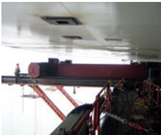
Cradle 13W getting pulled out from underneath westbound OBG
