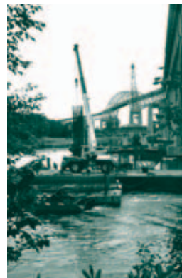
Work from Piers 1, 2 and 3, early September; on this day all cassettes were installed and Pier 2 columns completed; in the afternoon the cap form was set on Pier 2 and the rebar cages on Pier 1
