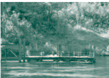
Pier one, all caissons were installed mid-August
