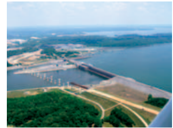
2005 to 2006 steel erection underway
