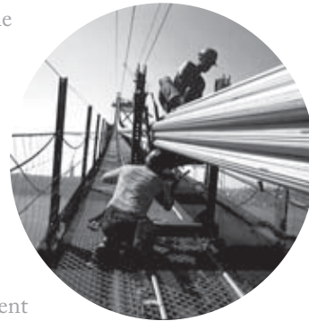
Controlled tension airspinning; still holds the efficiency record of 73 percent
