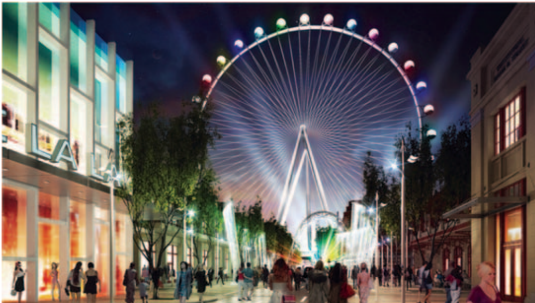
American Bridge Company's Special and International Projects District (SIP) is currently working on what will be the world's largest observation wheel when the project completes in late 2013.
