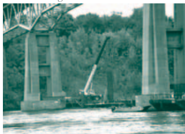
First rebar cage set at Pier 1
