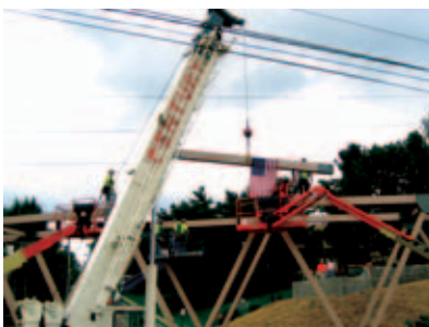
Field erection; ABM supplied the fabrication at cost, as did most of the suppliers
