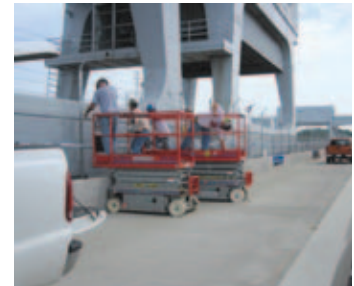
2010 to 2011 fence rehabilitation on existing dam/spillway
