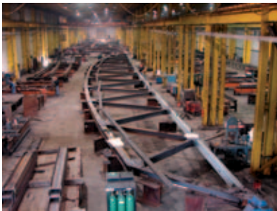
Truss fabrication at ABM's Coraopolis, PA shop
