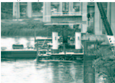
Setting the cap form at Pier 2, August 31
