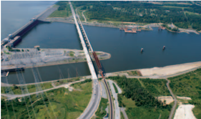
2009 traffic on new alignment
