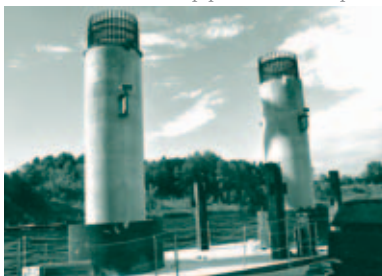
Columns at Pier 2, cap poured mid-September
