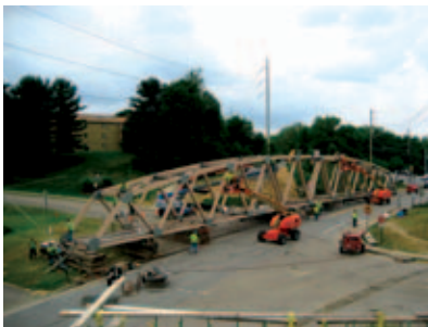
There were so many volunteers that the truss was erected on-site in two days
