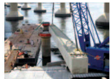
2011 setting precast for fishing piers
