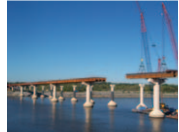
2007 to 2008 girder erection
