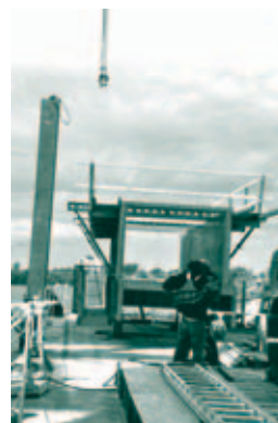
Cap form sits on the column seats; after all reinforcements were installed the concrete was poured, early September
