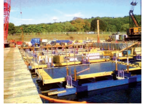
Concrete falsework deck
