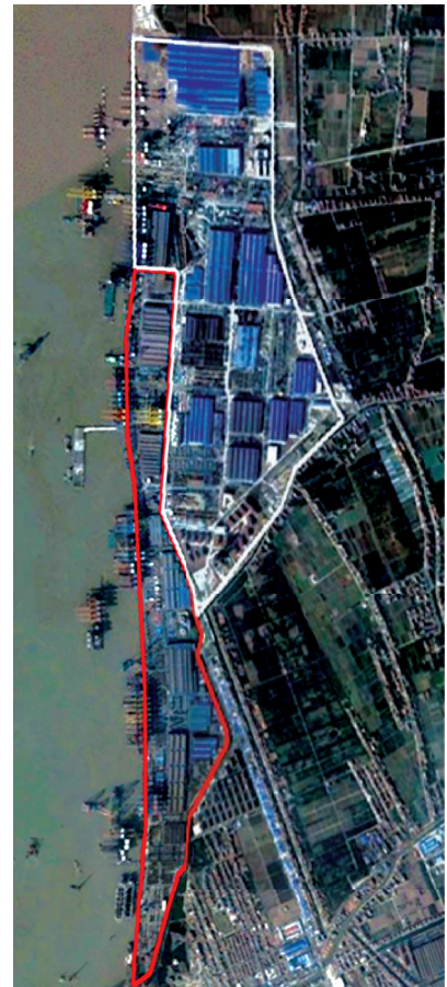
ZPMC Expansion since 2007 - red is the original base that was built in 2000 and the white is the expansion since 2007
