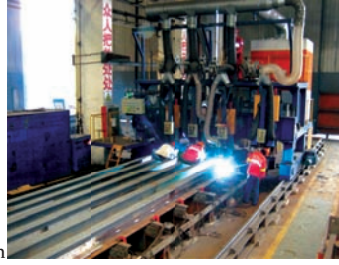
Side plate fabrication
