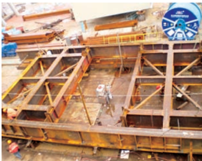
Cradles being fabricated - ABFJV puts the OBG lifts onto the cradles so they can be adjusted and welded together in Oakland
