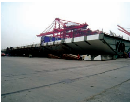
Side view of the trial assembly - full length is 525'
