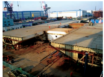
Trial assembly of OBG lifts 5 and 6 with the crossbeams connecting the east and west line of the bridge
