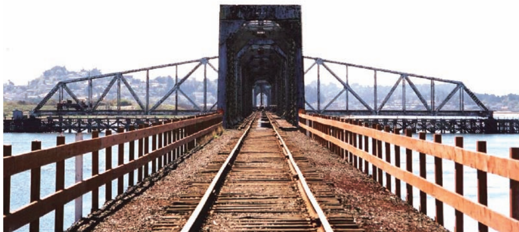
Coos Bay swingbridge, constructed by American Bridge in 1914, is part of the 111 mile Coos Bay Line closed in 2007. With funds from ARRA and a new grant, the line will be rehabilitated, restoring competitive advantage to ABM's Reedsport, Oregon plant.
