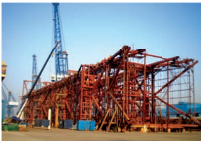
The erection tower being assembled
