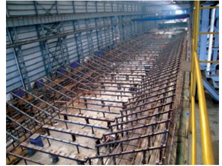
Segment assembly workshop before the plate layout has started showing the steel frame, called a jig - before any side or bottom plates can be put onto the jig, ABFJV surveys it and gives ZPMC the approval to start the segment assembly
