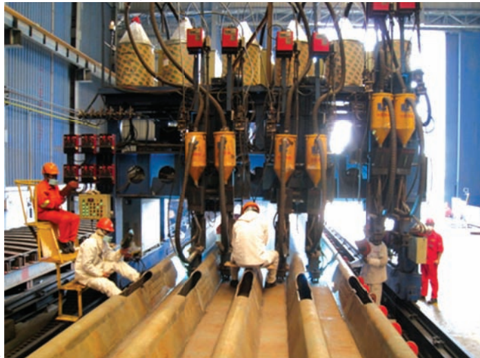
U-rib welding on the deck plate (for vehicular traffic) - U-ribs are set down onto the plate to a tolerance of 1/64" before welding to avoid a blowout (weld melts through steel) - since this is a closed rib and there is no access to the backside a blowout would cost ZPMC the whole deck plate
