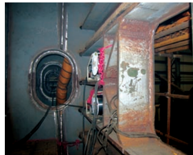
View from the inside of the mock-up - these manholes are located 12' above the bottom of the OBG
