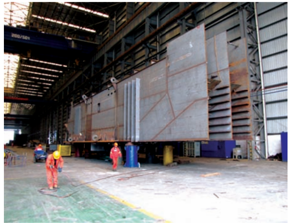
The east end mock-up of the OBG over pier E2 (400mt) which was completed to verify this section of the bridge could be fabricated
