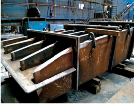
Saddle grillage - the point where the cable wraps around the OBG before it is anchored into the bridge
