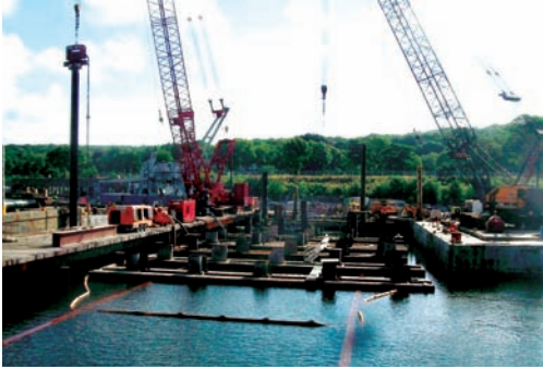
Pile driving operation from trestle and support crane
