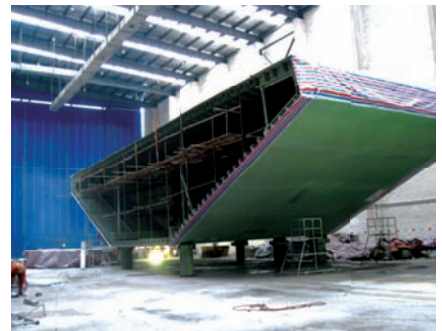
Painting the OBG - after painted they are moved to the trial assembly yard and welded together to lifts which consist of 2 to 5 segments and can be up to 210' long
