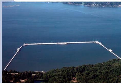
Overview of pier R3
