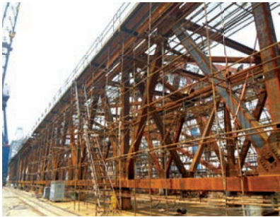
The full length of the trusses being vertically assembled was 800' and the dimension of the truss is 20' tall by 32' wide
