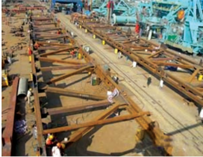
Trusses that currently carry the OBG and will continue to do so for the duration of the erection before bridge load is transferred onto the cable
