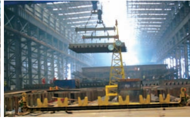
Lifting superpanel to segment assembly
