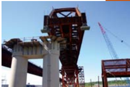
BEARINGS FLOATING OVER THE PIERS
