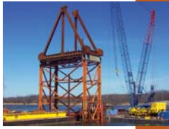
THE START OF THE PROJECT - 1ST PIECES OF THE TRUSS BEING ASSEMBLED
