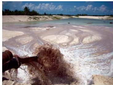
HYDRAULIC DREDGING TAKING PLACE
