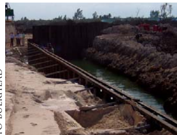
TIE-BACK ROD ANCHORS CONNECT THE DEADMAN TO BULKHEAD
