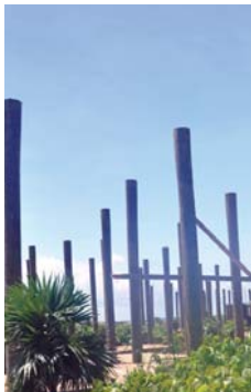
BEGINNING OF CABANA CONSTRUCTION
