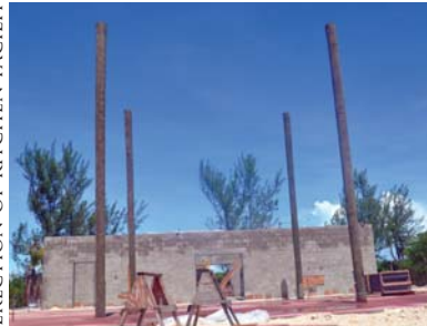
ERECTION OF KITCHEN FACILITY
