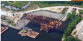
TRUSS ASSEMBLY ON FALSEWORK
