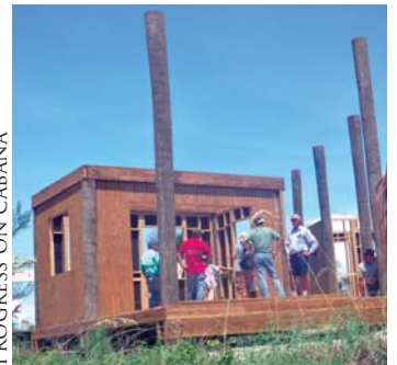
PROGRESS ON CABANA
