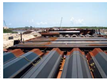
BALANCE OF AZ-13 SHEETPILE
