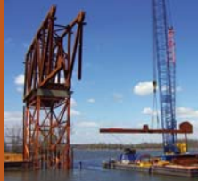
TRUSS BEING ERECTED ON FALSEWORK
