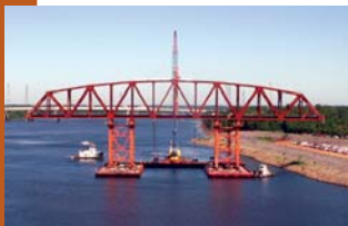
TRUSS FLOATING ON FALSEWORK IN THE LOWER APPROACH
