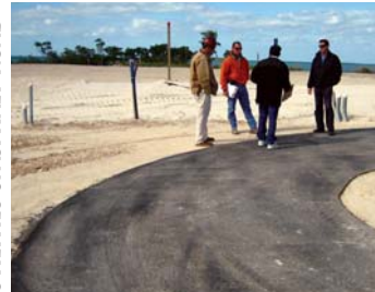
FINAL ELEVATION WITH UTILITIES & ASPHALT ROAD
