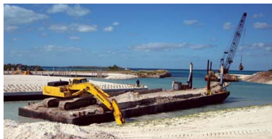
EXCAVATOR IN FOREGROUND; CLAMSHELL IN BACKGROUND
