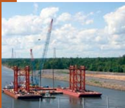
FALSEWORK ON BARGES AFTER THE BRIDGE HAS BEEN SET INTO PLACE
