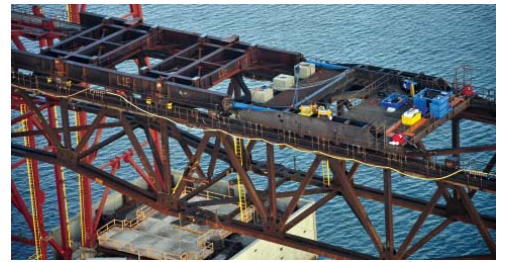
TEMPORARY TRUSS SHOWING ORTHOTROPIC BOX GIRDERS (OBG) CRADLE AND PUSHING FRAME. THIS WILL ALLOW THE OBG SEGMENTS TO BE TRANSLATED LONGITUDINALLY TO THEIR FINAL LOCATION
