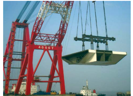
FIRST OBG TO BE LOADED ONTO SHIP
