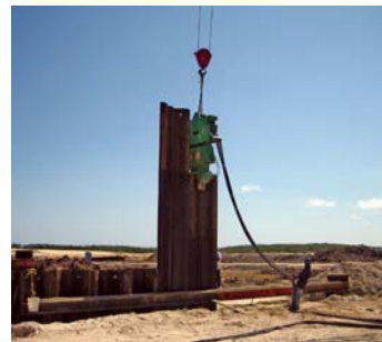
VIBRATORY HAMMER WEST ISLAND SHEETPILES
