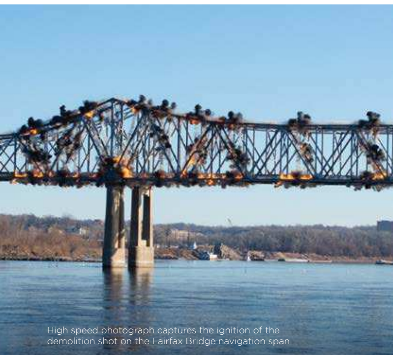
The navigation span of the Fairfax Bridge as it descends into the river
