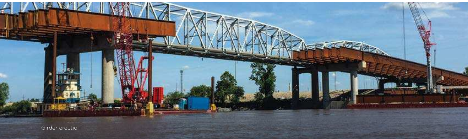
Girder erection utilizing a two crane pick over the navigation span
