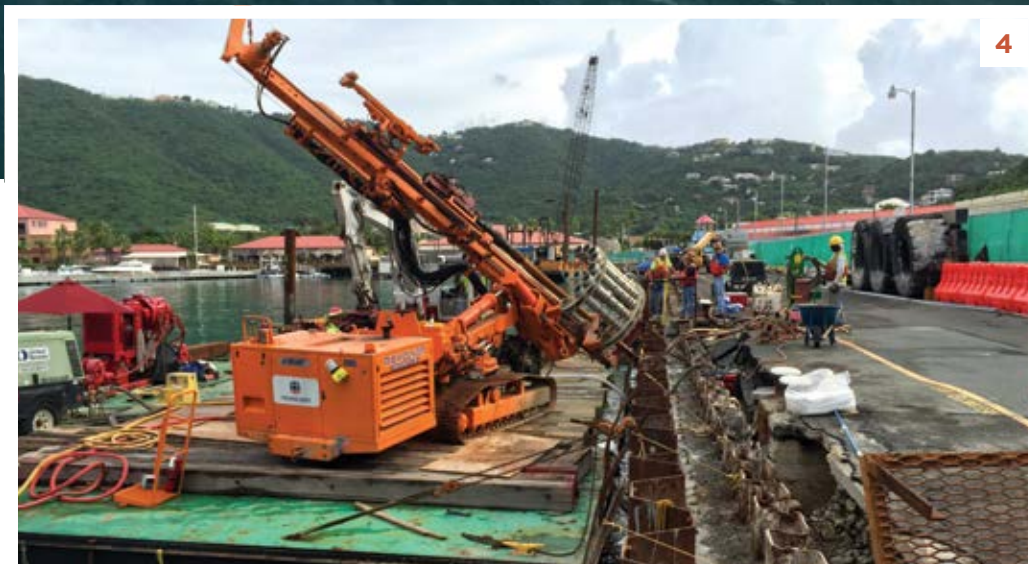
Photo 2: Cruise ship tying off to the newly installed SB-150 Bollards; Photo 3: Cruise ship tying off to the newly installed MT-150 Bollards; Photo 4: Looking east on the WICO dock as AB supports Nicholson (subcontractor) in drilling the holes for the permanent soil anchors
