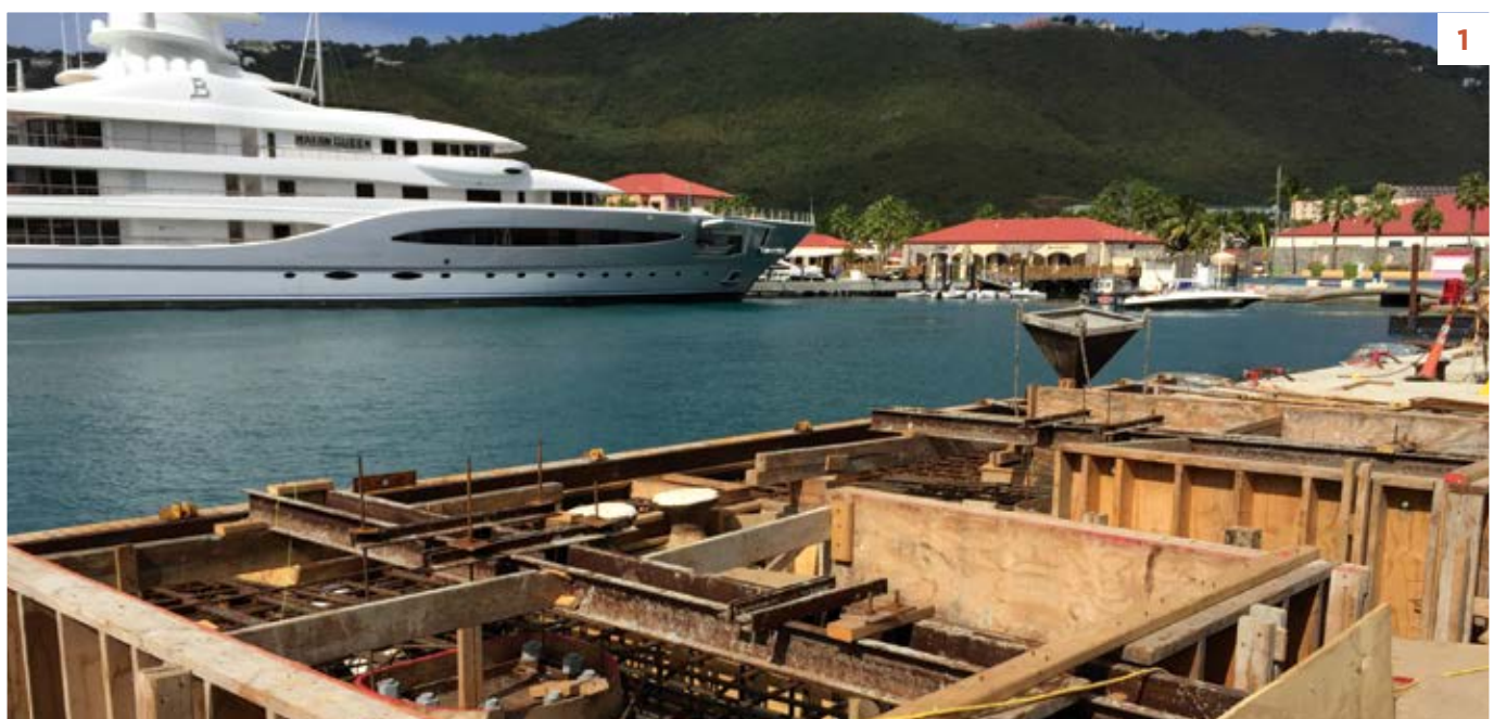
Photo 1: Wood formwork, rebar cages, as well as the EFCO forms and bulkhead rebar in place to support a double bollard and bulkhead concrete pour
