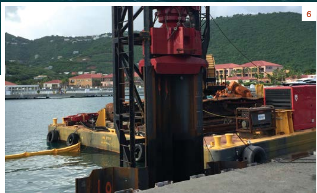
Photo 5: American 9310 moving sheetpile onto the barge; Photo 6: Impact hammer being used to push down a pair of sheet piles
