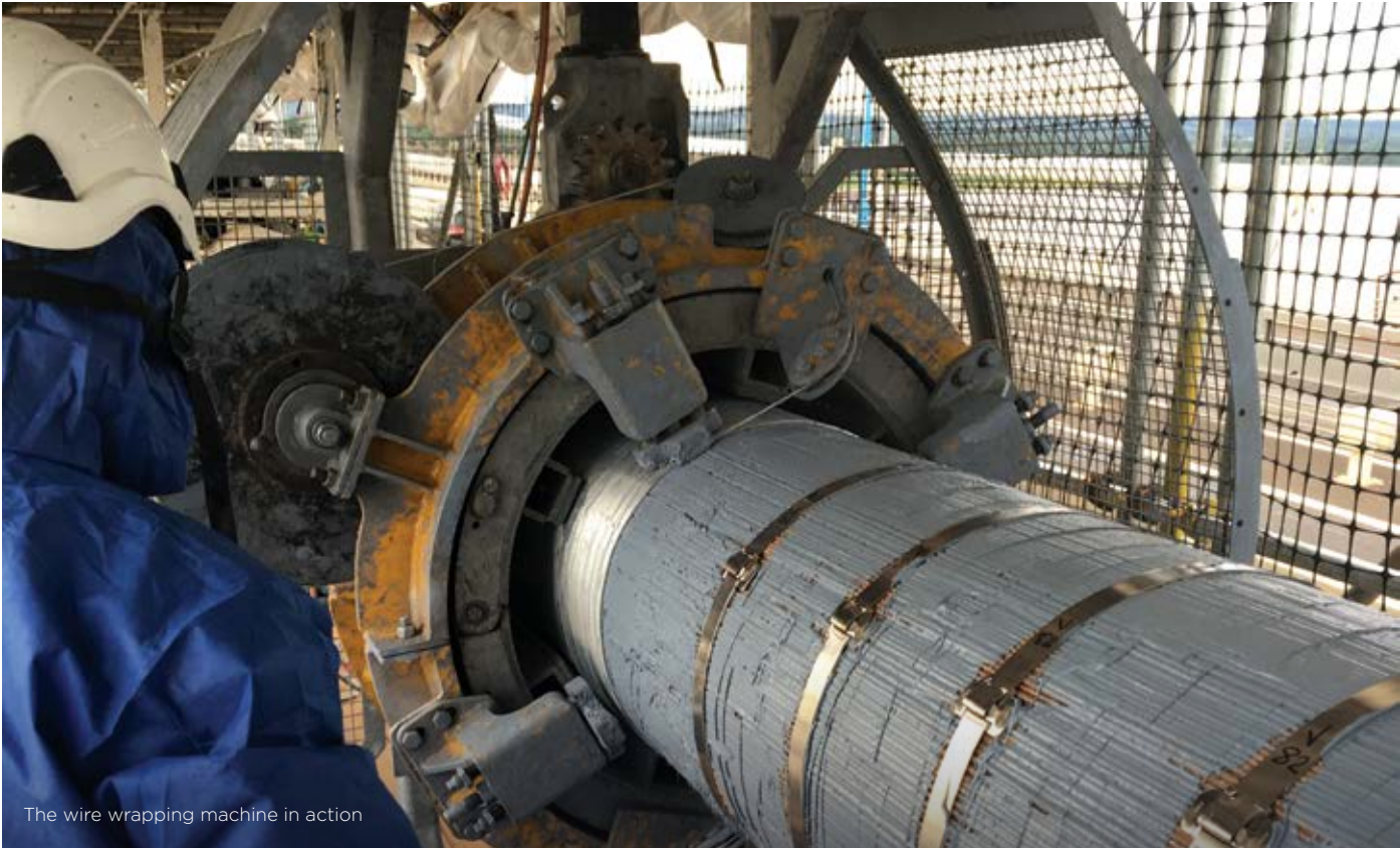
Inspecting an open wedge line
